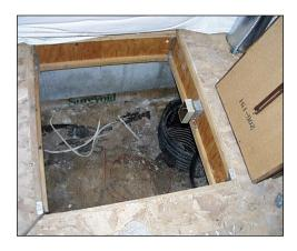
Some crawl spaces have humidity and temperature sensors that turn ventilation fans on and off. Do not set the humidity sensor above 40% relative humidity (RH) or the thermostat below 40°F.
