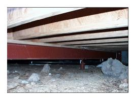
A ground cover (10 mil plastic sheeting or equivalent puncture- and moisture-resistant material) can help control a moisture problem in your crawl space. It is best for the ground cover (also called "vapor retarder") to be completely sealed to the
